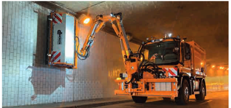
Use of TWA in the tunnel
