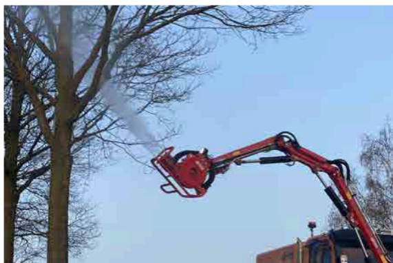
Blower with spraying device in use
